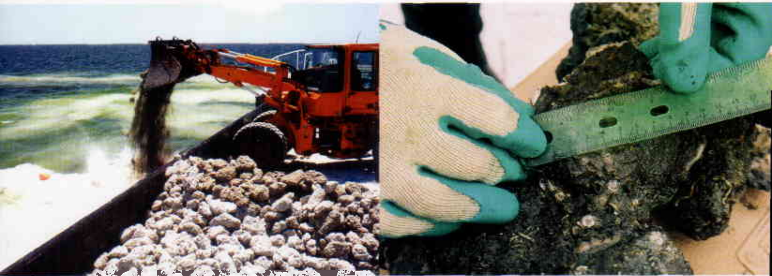
Figure 2: Limestone marl has successfully been used to create oyster reefs in North Carolina's Pamlico Sound (Ashley Harraman, TNC; Rob Brumbaugh, TNC)
